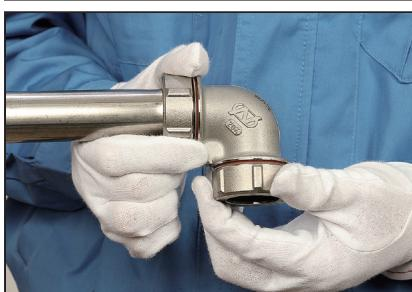
8. Set the conical washer to a section where the cap nut side surface comes in contact with the fitting and tighten the nut until the colored surface is not visible.
