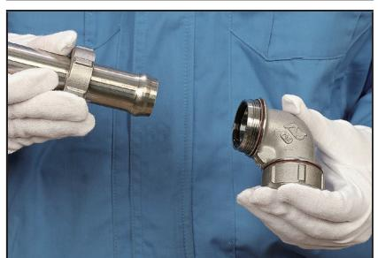
6. Insert the enlarged pipe into the fitting and tighten the cap nut.
